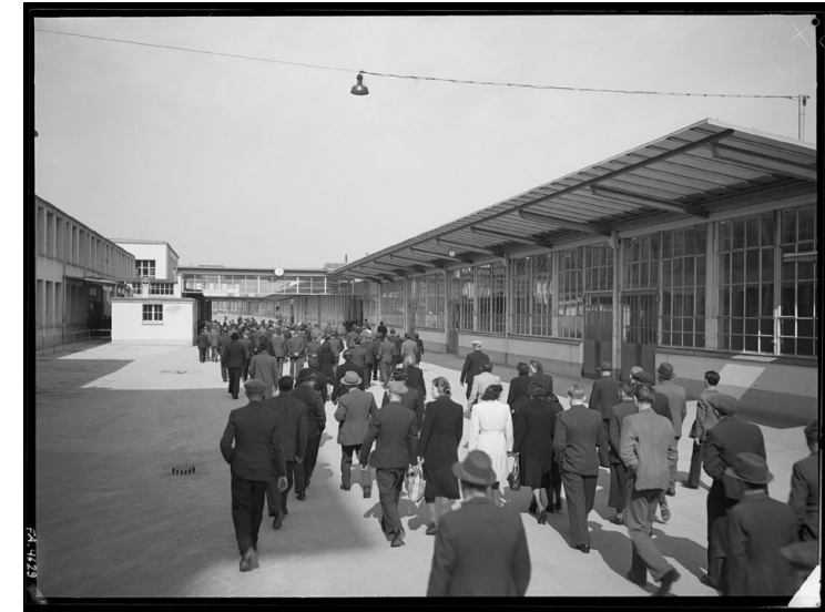
Staff of work at the Landis & Gyr plant in Gubelstrasse
